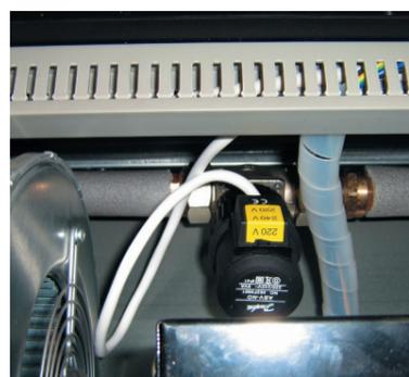
Built-in thermoelectric valve controls temperature of exhausted or spatial air.
