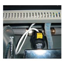
Built-in thermoelectric valve controls temperature of exhausted or spatial air.
